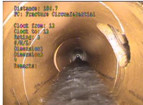
MH 195-194: Circumferential Cracking at Lateral
