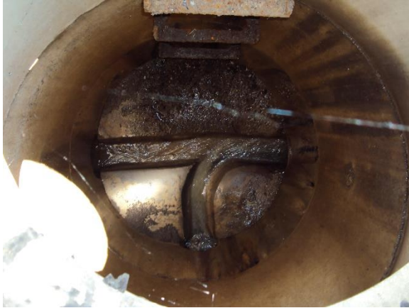
MH 144: Infiltration at Joints, Lifting Holes, Invert Needs Patched
