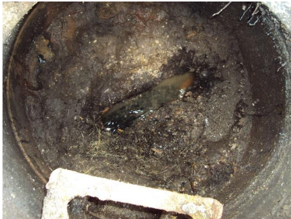
MH 194: Full of Debris, Roots, Joints Leaking
