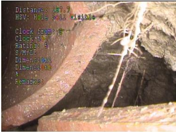
MH 142-141: Break in Pipe near MH 142
