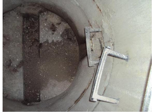
MH 140: Rings and Casting Offset, Full of Debris and Needs Adjusted to Grade
