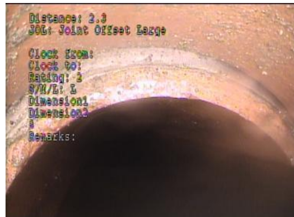
MH 151-152: Joint Offset near MH 151
