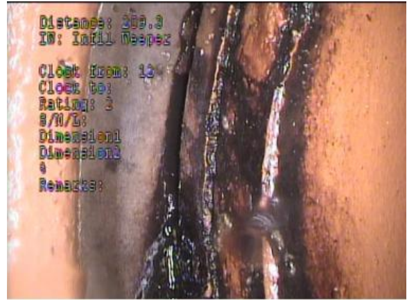
MH 145-144: Leaking at Joint
