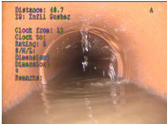
MH 153-148: Infiltration at Joint
