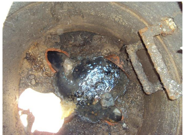
MH 148: Buildup in Invert, Signs of SSO's
