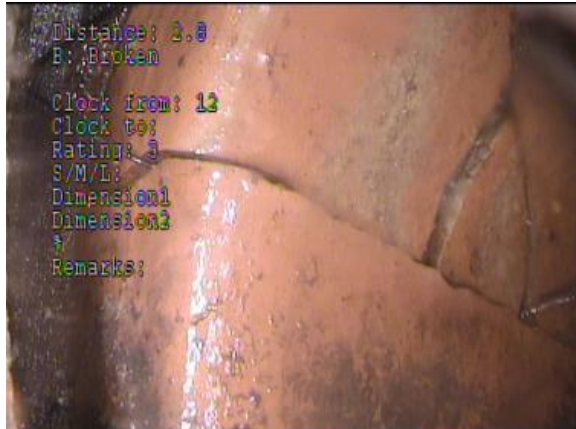
MH 146-147: Break in Pipe near MH 146
