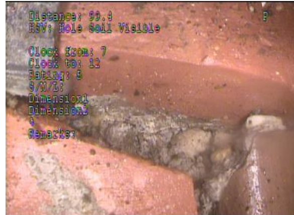
MH 150-151: Break in Pipe 100' from MH 151
