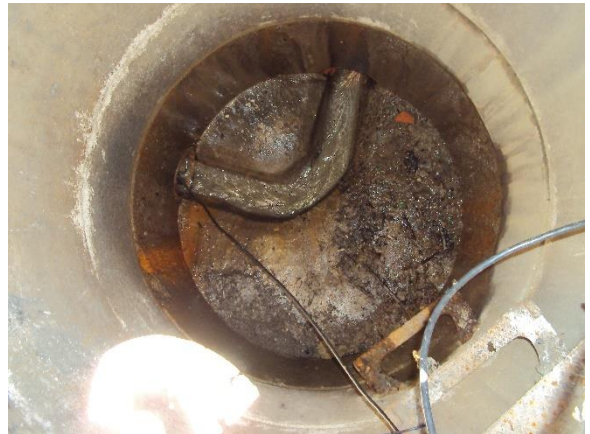
MH 147: Infiltration at Barrel Section
