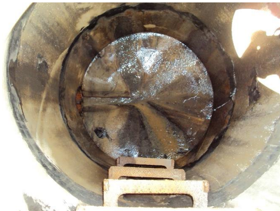
MH 145: Major Infiltration at Joints Leaking
